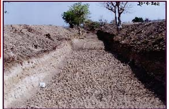
Structures across Gradient of Nala Bed to reduce High Velocity of Runoff Rain Water flowing in the direction RIDGE to VALLEY
