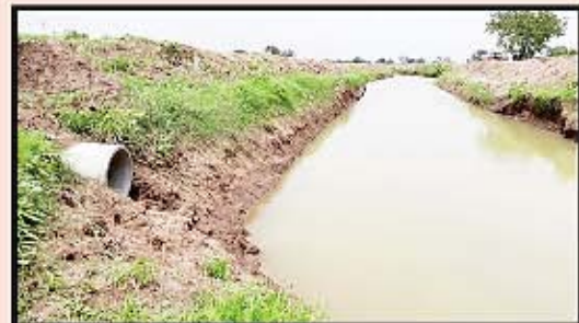
Rain Water Storage - 7 July 2017
