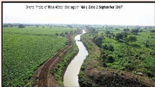
Drone Photo, Storage - 2 September 2017
