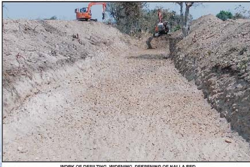
WORK OF DESILTING, WIDENING, DEEPENING OF NALLA BED
