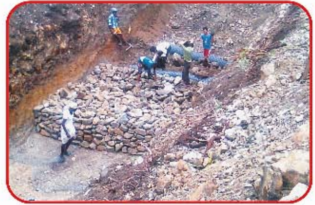
Gabion Bandhara Using Local Material
