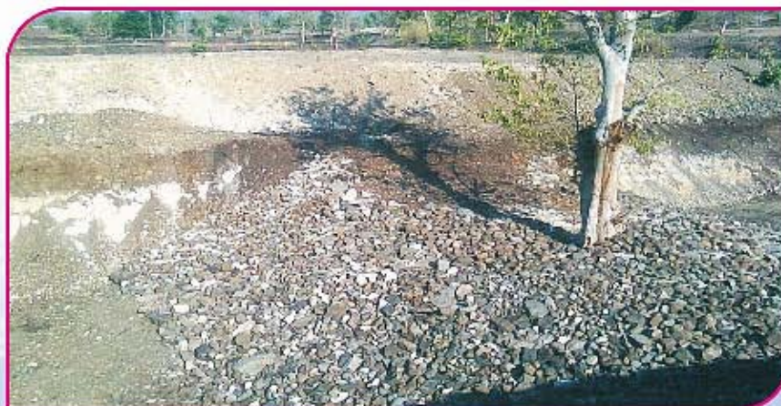
EARTHEN BANDHARA STONE PITCHING (TO REDUCE HIGH VELOCITY) 500 MT POINT
