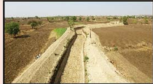
Treatment Work - May 2017
