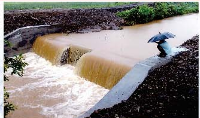
No Flood as excess Water goes to next Compartment Gradually to fill Compartment towards Valley portion.
