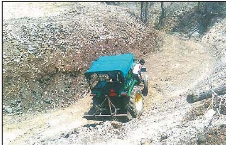
WORK OF DESILTING, WIDENING, DEEPENING OF NALLA BED
